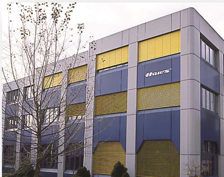
EMEA Headquarter Burgdorf, Switzerland
